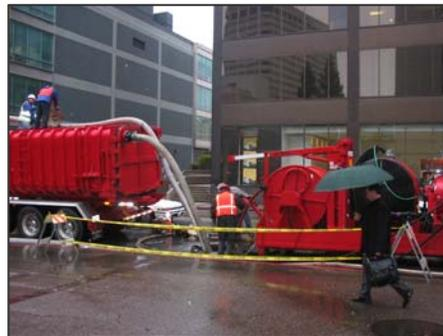
*Sewer Hog™ and Grit Gator (dewatering box) were set up near 20th Street and Broadway.*
