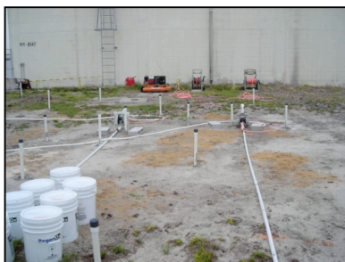
NASA's Vehicle Assembly Building (left), about 400 yards from Launch Equipment Shop, was the world's largest building when completed in 1962-65. Tetra Tech used re-injectable wells (left and center) to emplace RegenOx™ into contaminated soil and groundwater behind the LES.
