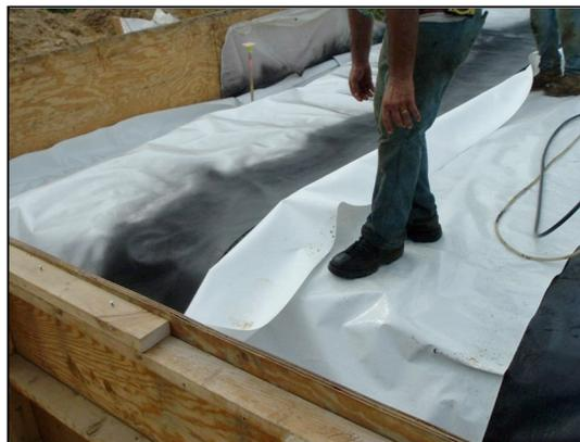
*Triple-layer Geo-Seal™ system includes two chemical-resistant bonded HDPE layers enclosing an elastic, copolymer-modified asphaltic membrane core. The core is spray-applied, creating a highly effective seal around piping and other slab penetrations and eliminating the need for mechanical fastening at termination points.*
