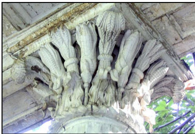
(top) Litchfield Villa in 1963; (bottom) columns are an American order, featuring corn and wheat motifs.
