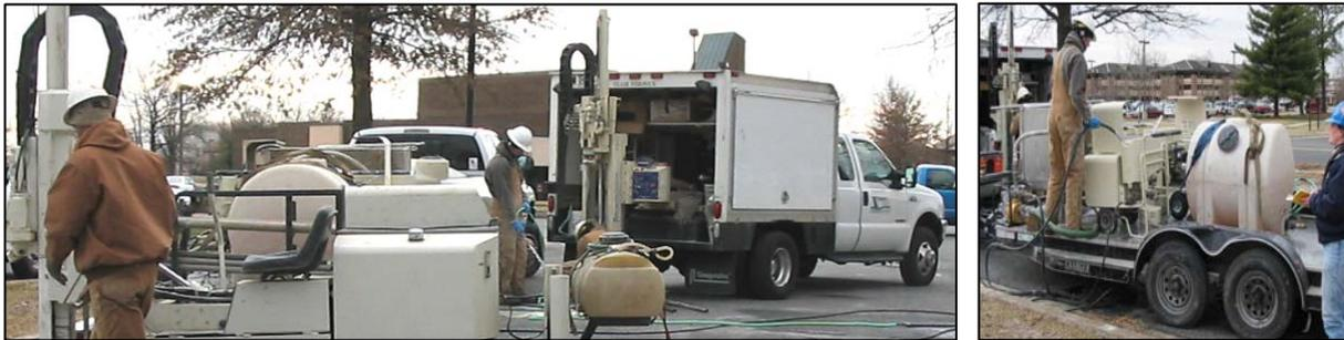
*Following removal of saturated soils from source area, five-acre contaminant plume at Andrews AFB was remediated in-situ by injecting ORC Advanced™ into the subsurface, using conventional, self-contained direct-push equipment.*
